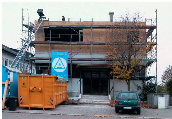
Figure 10.2-2 The construction of the second story on the building in Tullastrasse 2
