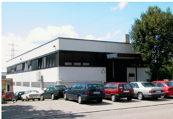
Figure 10.2-1 Halle 1 in 1999 before building work started on the first floor
