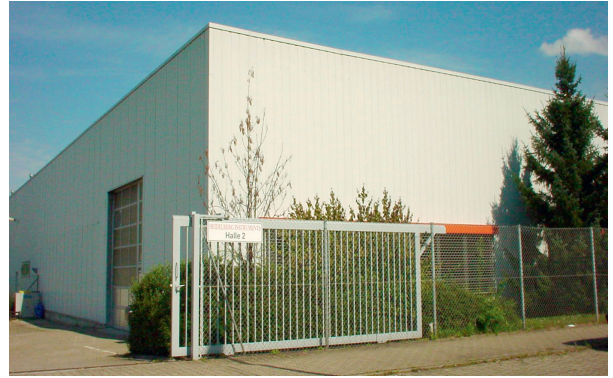
Figure 10.1-1 The Old Halle 2, which around the turn of the millennium was used for the assembly of PCB systems and very large systems (image shows the entrance to Heidelberg Instruments’ part of the building on Hatschekstrasse).
